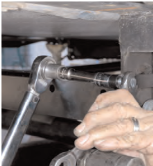
Install and torque the crossmember bolts.
